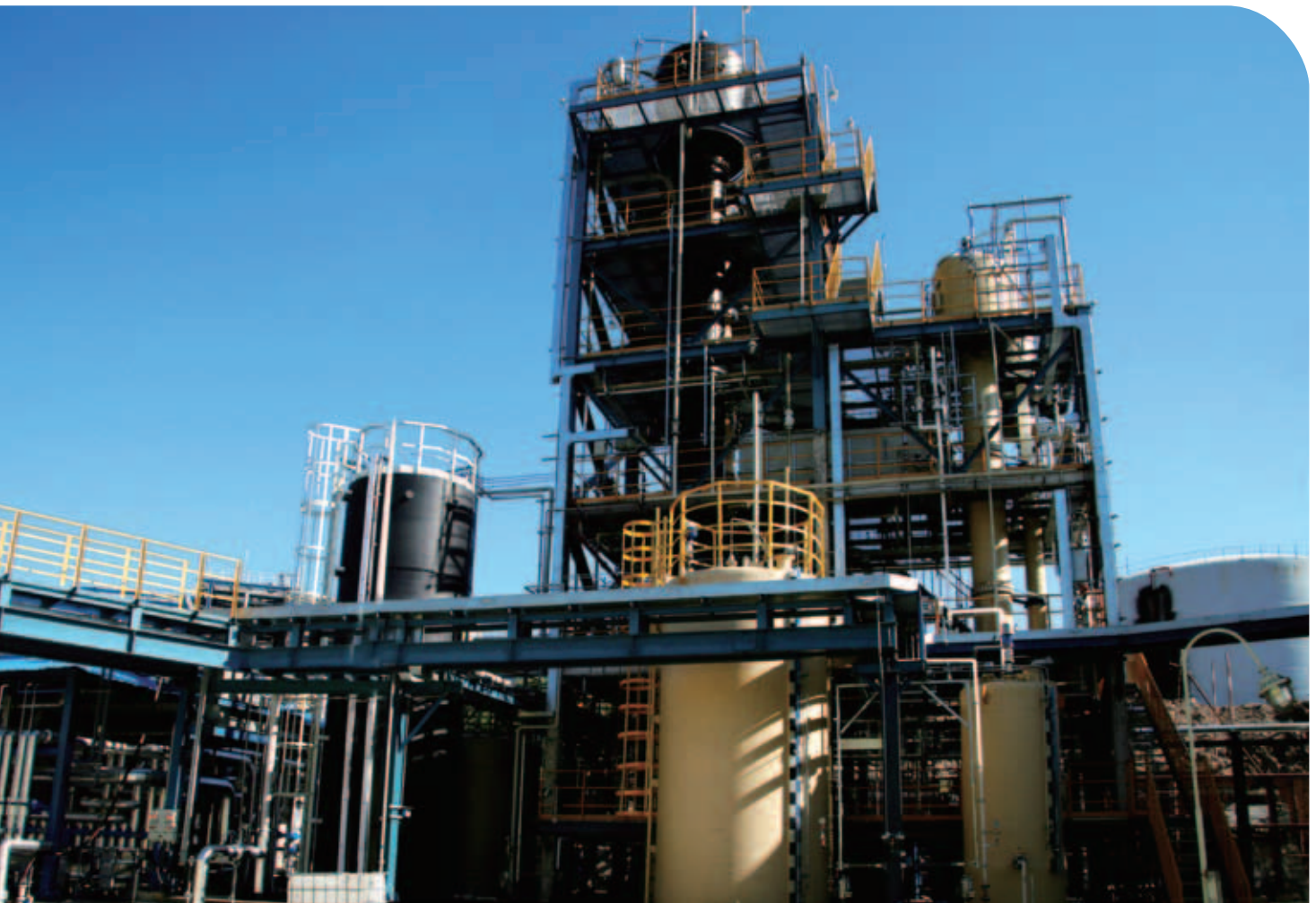
The world's first bromine extraction facility, LLX columns
